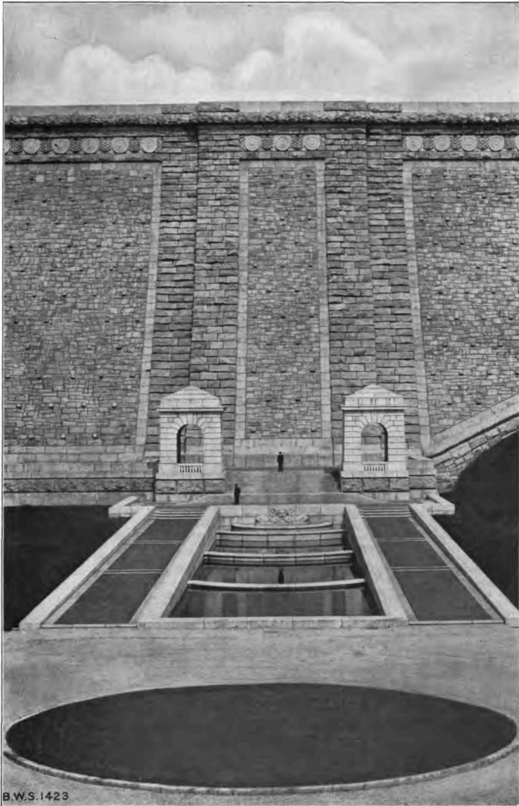
KENSICO DAM—The East pylon and cascade basin showing details of the architectural design and the rugged character of the stonework in keeping with the massiveness of the structure.
