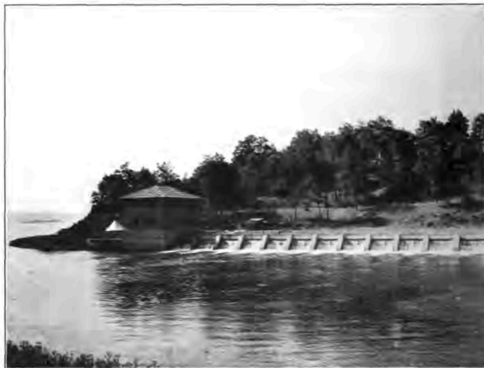
KENSICO RESERVOIR—Kensico Influent chamber and weir, at the northern extremity of the reservoir. The weir is formed by a slot in the aqueduct arch over which the water flows when gates in the Influent chamber (down-stream) are closed. To divert the aqueduct flow from the reservoir, the gates are opened and the water flows through Kensico by-pass
