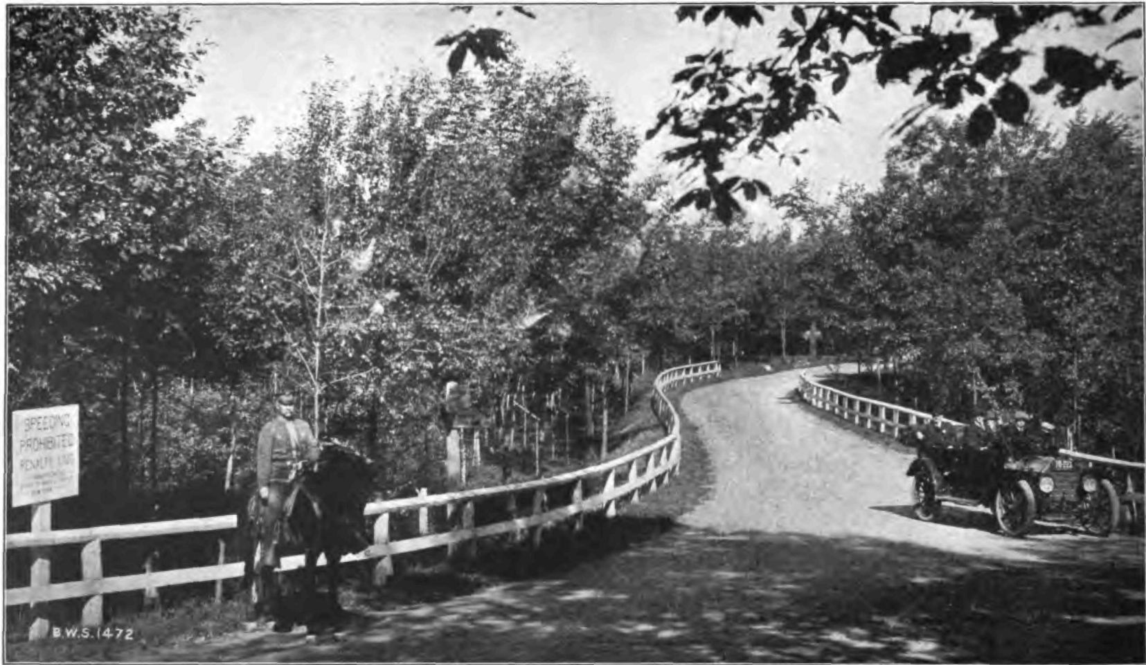
ASHOKAN RESERVOIR—Substituted new highway, Road 20, looking easterly, at its junction with Tongore highway. Note Board of Water Supply Police officer and "Speeding" and Direction signs
