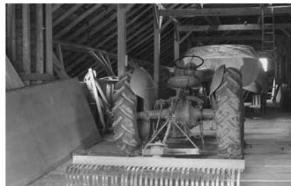
The top floor of the barn is accessed from the ramp over the road and allows for the wagons to be emptied at the top of this ingenious hay mow. The top of the side-storage bins can be seen to the left of the tractor.
