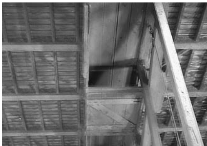
Do not look over the edge of the floor at the top of the barn if you have a problem with heights. Here, you can see storage area for the loose hay, and at the far side is one of the chutes by which hay can be dropped from the top of the mow straight down for nearly 100 feet to the cows in the basement.
