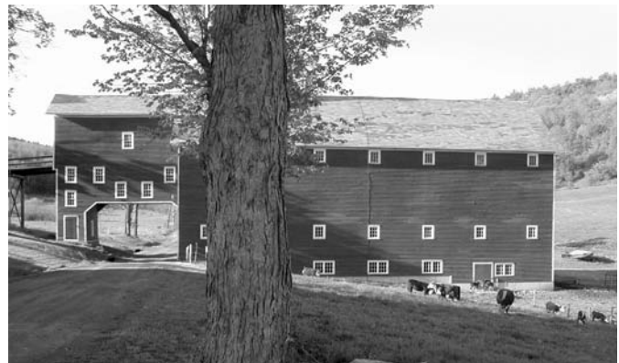
The Decker-Starheim barn has been completely renovated for the twenty-first century but retains the imprint of its nineteenth-century beginnings.
