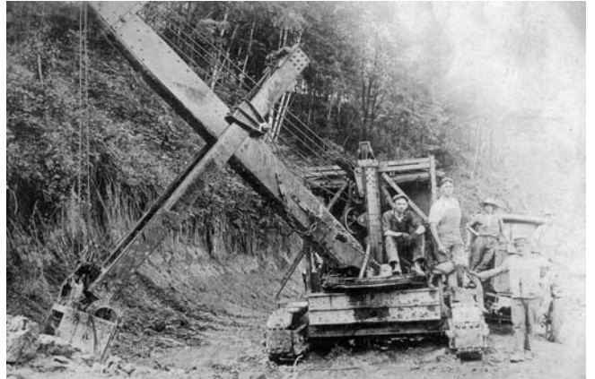
Other early equipment was a steam shovel (yes, driven by steam) next to the Lynn tractor (above) and a crane (below).
