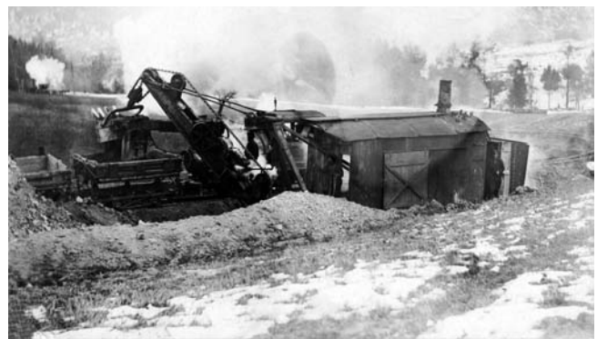
While we are not certain, the terrain suggests that the steam shovel in this view is working Clay Hill behind the Hardenburgh House in the Town of Roxbury. After leaving the cut at Clay Hill, the railroad crossed Bear Kill at Hardenburgh Falls, north of which a short tunnel was planned. (Richard F. Makse Collection)
