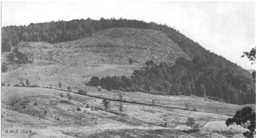
Site of the Stevens Mountain quarry had been cleared in 1920. This hill (to the east of the current Gilboa-Conesville Central School) provided the crushed stone for the concrete used in the construction of the Gilboa Dam. Grading of Road 1 (a.k.a. State Route 990V) is shown in foreground. Photo courtesy of the NYC Bureau of Water Supply's Annual Report for 1920.
