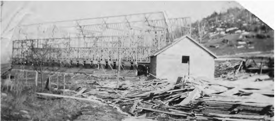
The beams and some of the 2 × 4s were in place for the second-floor walls when a windstorm came through on March 23, 1923. By late spring, the mess was cleaned up, more 2 × 4s and the roof were put in place, and shingles were being placed on both the west side (below) and east side (bottom). The east side had entrances for two bridges to allow hay wagons into the hay mow.
