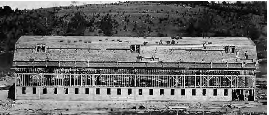
The beams and some of the 2 × 4s were in place for the second-floor walls when a windstorm came through on March 23, 1923. By late spring, the mess was cleaned up, more 2 × 4s and the roof were put in place, and shingles were being placed on both the west side (below) and east side (bottom). The east side had entrances for two bridges to allow hay wagons into the hay mow.
