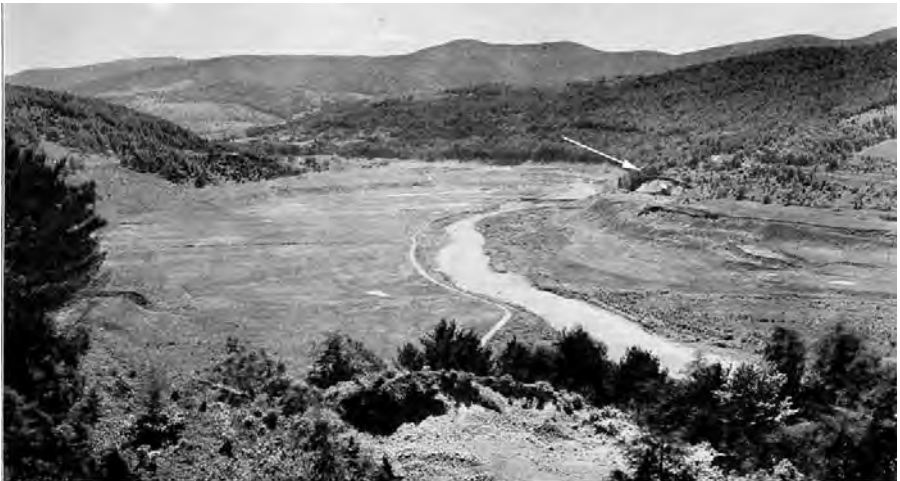
1925. Part of the Schoharie valley to be flooded by the waters of the reservoir, looking to the south from a point above the Manor Kill. The reservoir basin has been cleared of trees and the steep slopes grubbed to elevation 1135 using generally local labor. The temporary bridge across the creek was used by another narrow gauge railroad that brought sand from the Patchin Pit to the mixer. The gatehouse and intake chamber of the Shandaken Tunnel is hidden in the trees (arrow) just past the railroad. Photograph scanned from the Annual Report of the Board of Water Supply for 1925 , used courtesy of Department of Environmental Protection.
