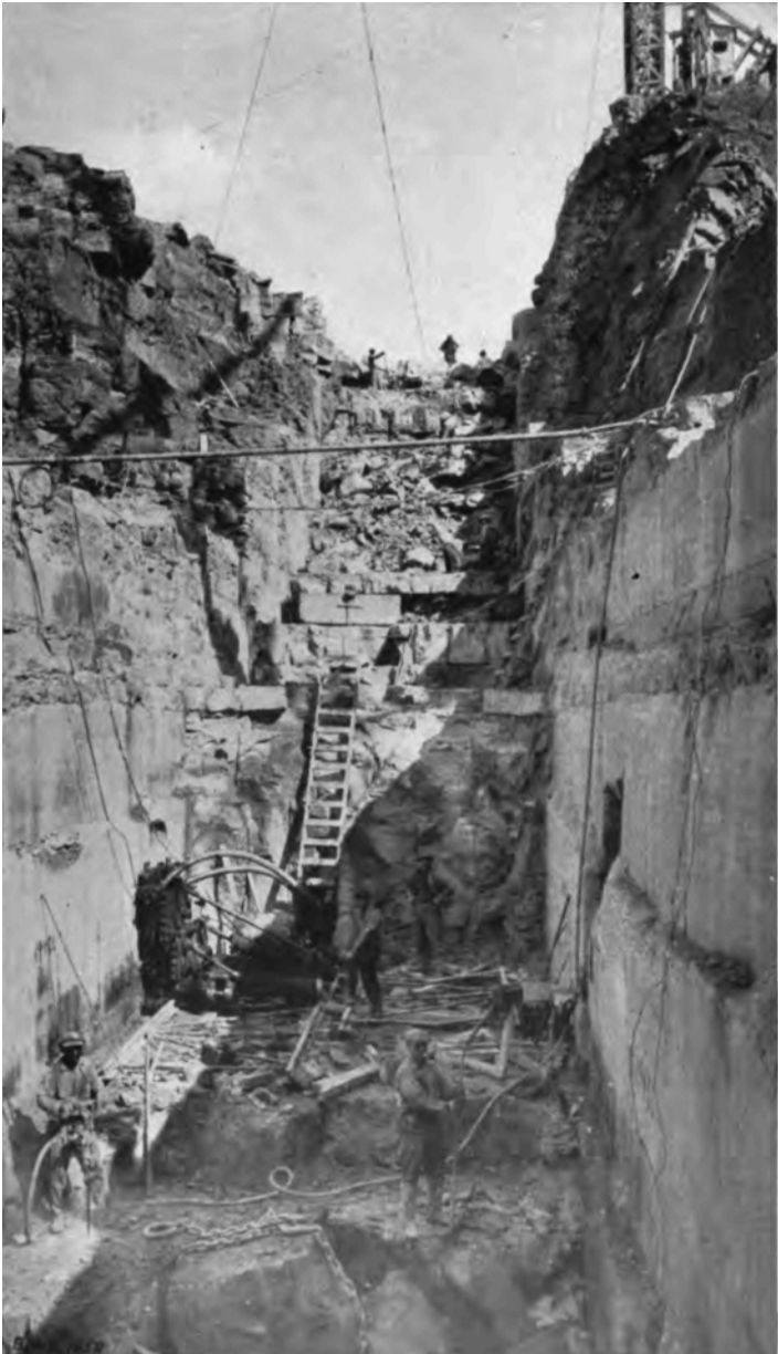
1921. The first step is construction of a cut-off trench to excavate all permeable material so that water can't seep under the dam. This is looking east along the excavation for the cut-off trench. The bottom of the cut-off is at elevation 949. Photograph scanned from the Annual Report of the Board of Water Supply for 1921 , used courtesy of Department of Environmental Protection.
