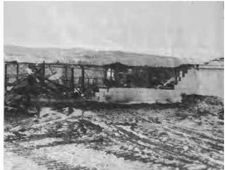
Only concrete and twisted steel remaining of the leveled Prospect Farm dairies barn following Monday night's fire. Photograph courtesy of the Mirror Recorder , Stamford, New York January 31, 1968 from the scrapbooks of Norma and Claude Cooke
