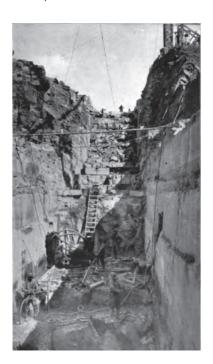
Excavation (cut-off) for the dam foundation looking to the east. The bottom of the cut-off is at elevation 949 feet, the approximate depth of cut-off trench is 35 feet, and the top of the dam is projected at 1135 feet.
