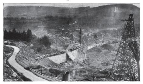
SCHOHARIE RESERVOIR—View of the Gilboa dam from bank along Road 8, looking easterly across the core-wall of the earth dike and the masonry portion of the dam. The track for transporting embankment material from the borrow-pit to the bank is shown at left with the switch-back to the top of the finished core-wall. Courtesy of DEP Archives
