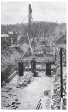
Left: There is a construction crane placed on top of the dam, and to gain added height, the crane was built on three stilts. These stilts were made from the 9-foot-diameter pipes that had previously been used to carry water between the 2 coffer dams.
